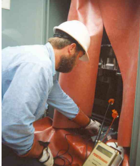
Fig 15 – Use of insulating mats in switchboard application
